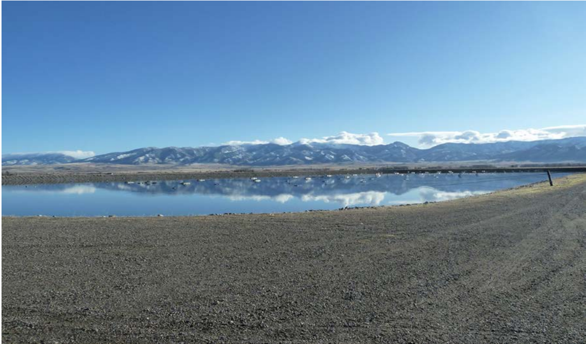
Belgrade Waste Water Treatment Facility adjacent to BZN
