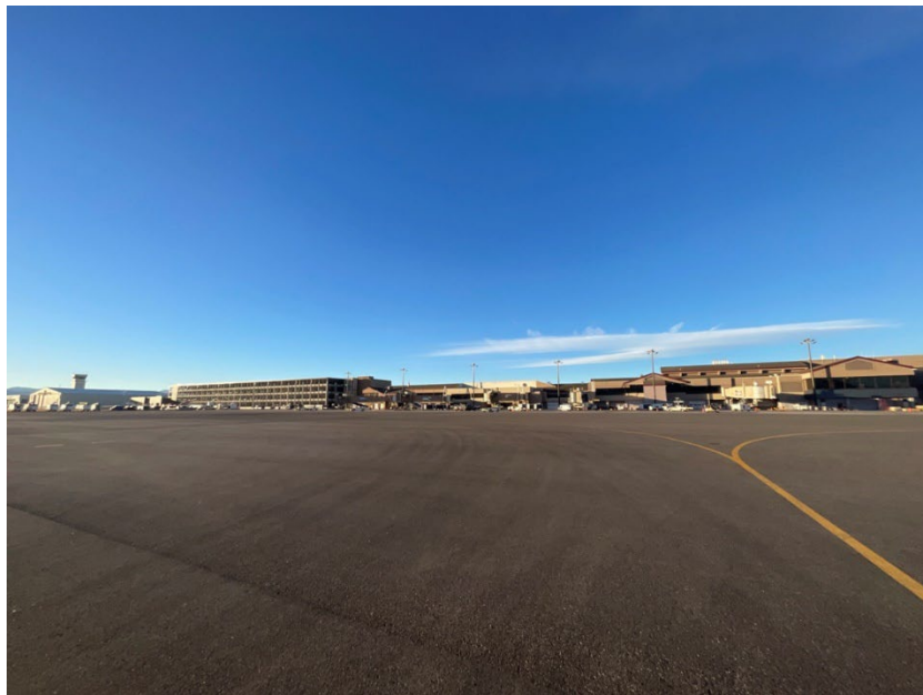
Figure 6.57. 24GA2343, overview showing the modern parking structure to the left, the 1977 terminal in the center, 1996 expansion to the right.
