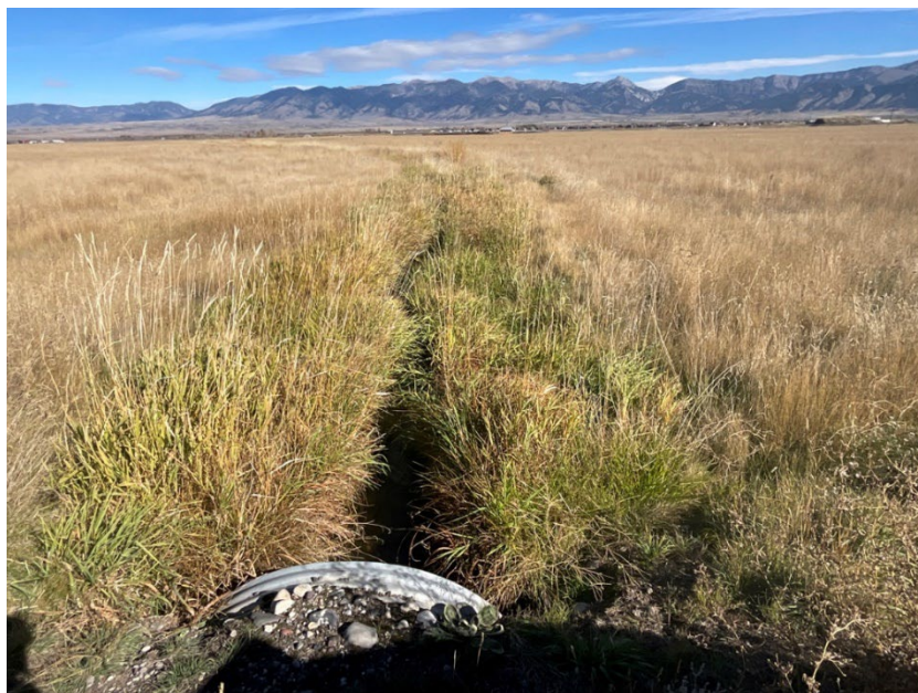
Figure 7.3. 24GA0741 at the AARF Road, northwest end of Runway 12-30, view to the north.
