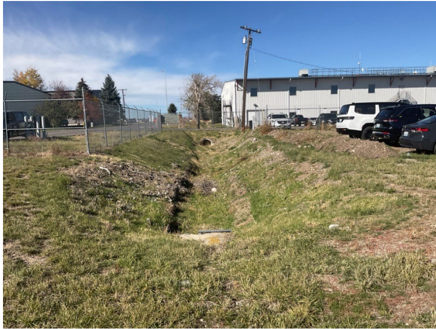
Figure 7.11. 24GA0743 abandoned segment at Taxiway “H,” view to the east.
