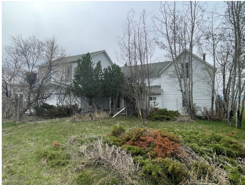
Figure 7.25. 24GA2327, north elevation, view to the south.
