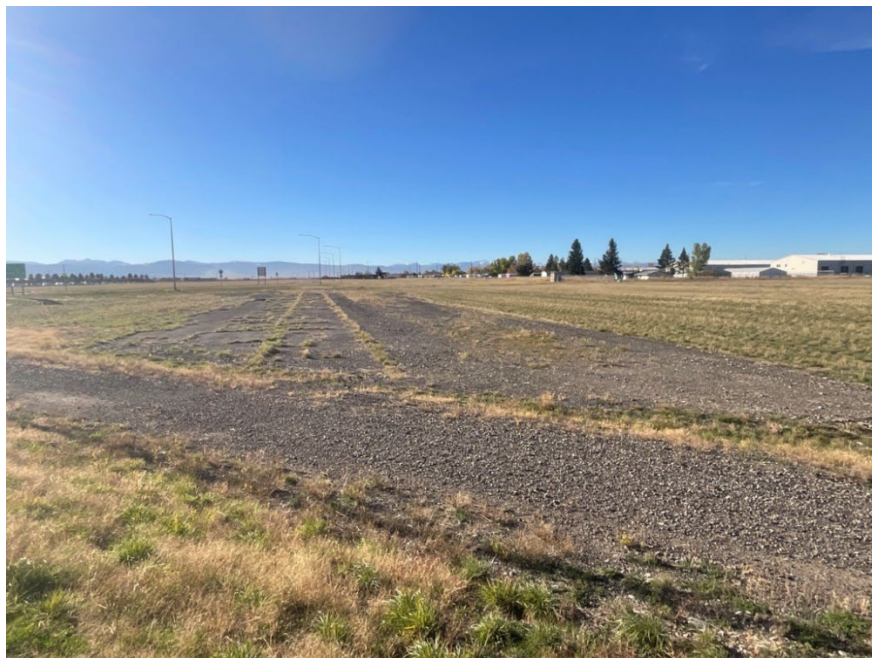
Figure 6.28. Runway 16-34 near its intersection with Airway Blvd., view to the south from Airway Blvd.
