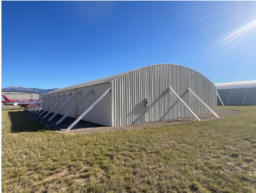
Figure 6.43. 24GA2320, Hangar 9, west corner, view to the northeast.
