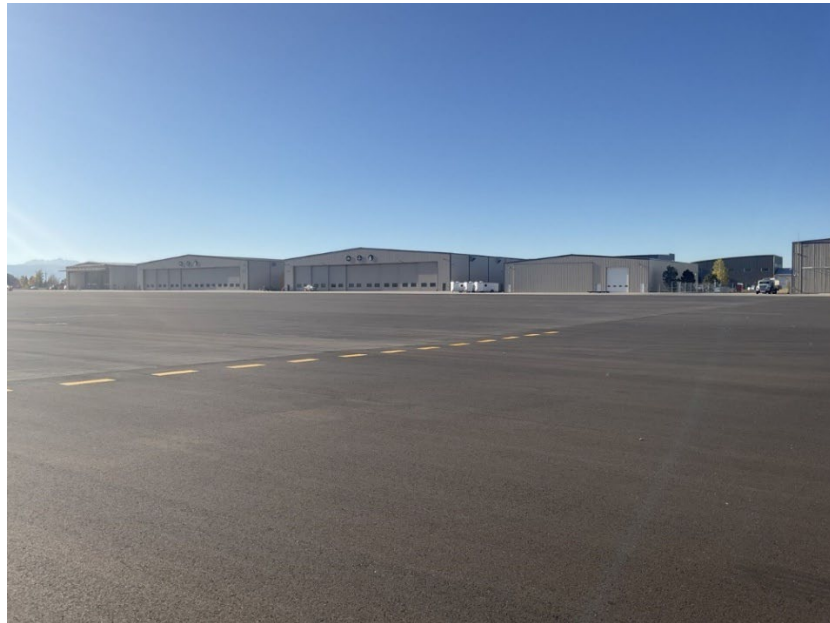
Figure 6.2. East Apron front line, view to the south.
