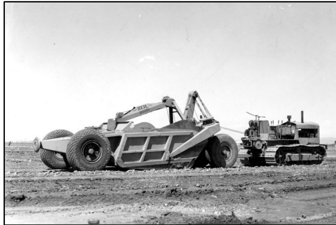
Figure 3.3. Runway grading in 1942, photo courtesy of the Gallatin History Museum, Photo 39.
