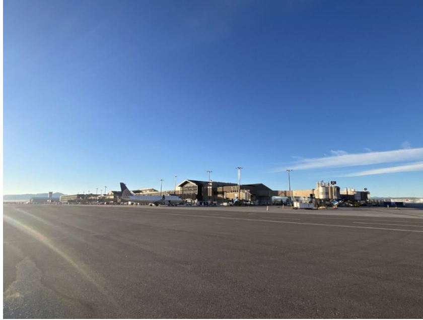
Figure 6.10. Western end of the modern terminal from the Terminal Apron, view to the southeast.
