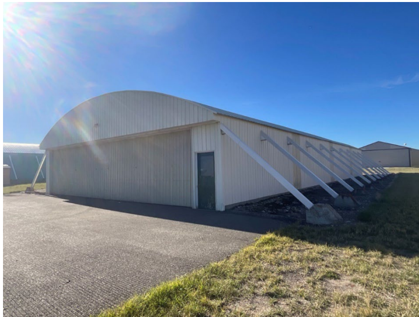
Figure 6.42. 24GA2320, Hangar 9, north corner, view to the south.
