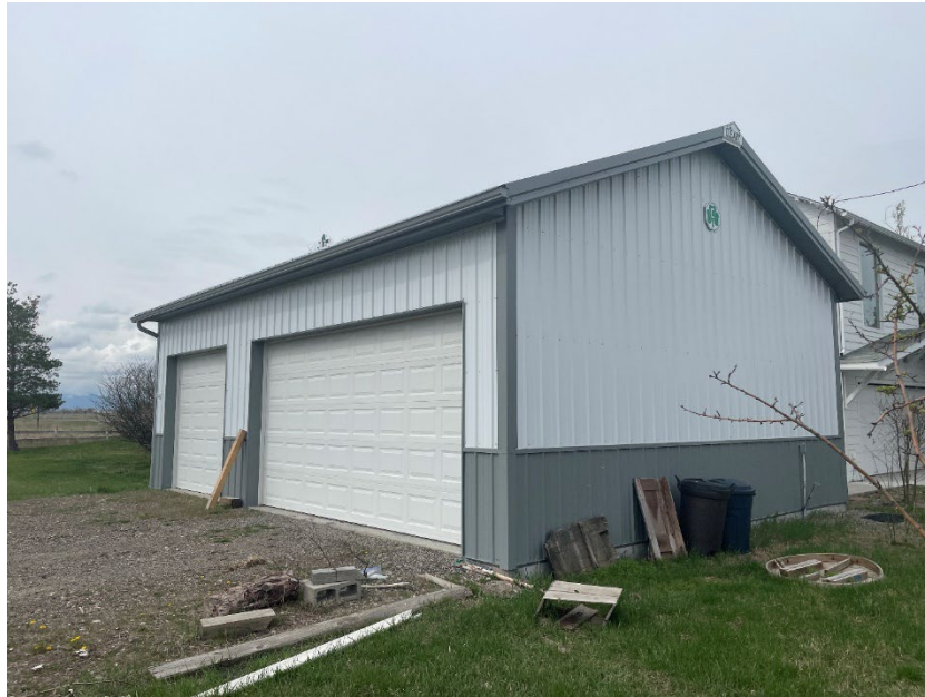
Figure 7.26. 24GA2327, modern shop, northeast corner, view to the south/southwest.
