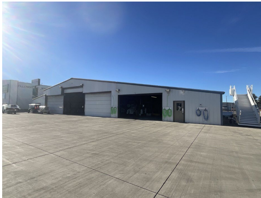
Figure 6.11. Hangar 5 on the front line of the GA Apron, view to the south.
