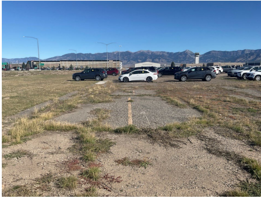
Figure 6.27. Taxiway “B” near its intersection with Airway Blvd., view to the north.
