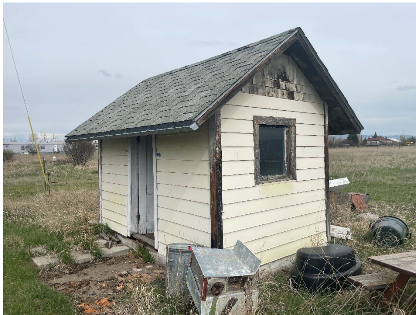
Figure 7.27. 24GA2327, gabled storage shed, view to the northwest.
