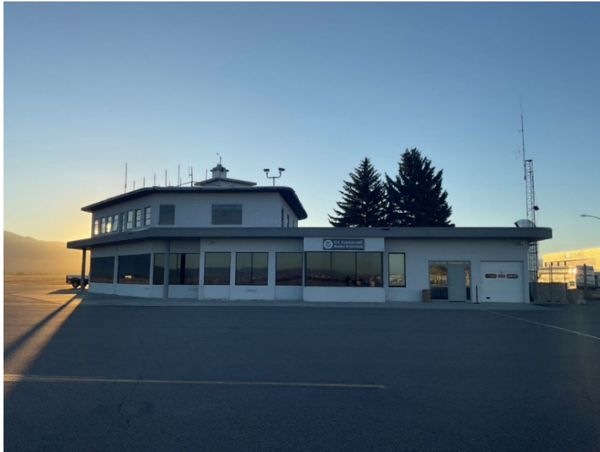
Figure 6.23. 24GA1654, northwest elevation, view to the southeast.
