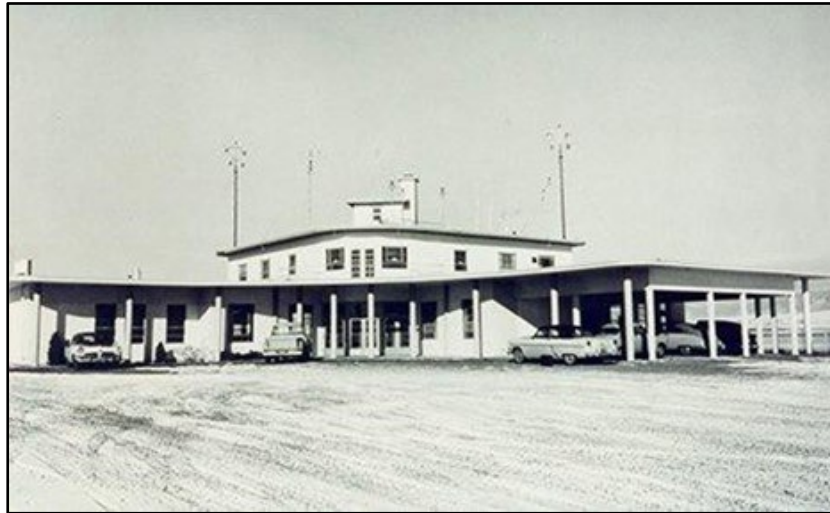
Figure 3.6. BZN Terminal and Flight Service Station, ca. 1952 (MMI 2020:1-5).
