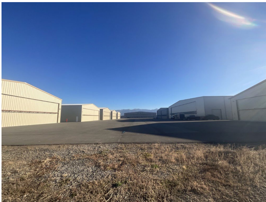
Figure 6.4. Modern hangars at TLY South, East Apron, view to the north.
