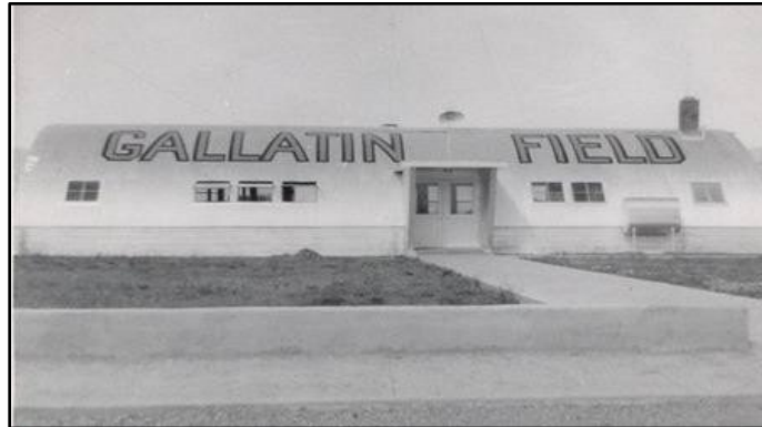
Figure 3.5 Gallatin Field temporary depot for Northwest Airlines, ca. 1948 (MMI 2020:1-3)
