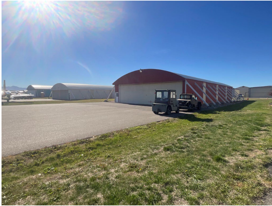
Figure 6.39. Overview of Hangars 8-10 from Hangar 10. View to the east.
