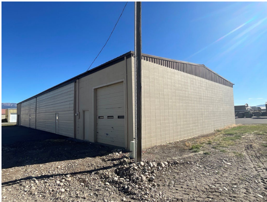
Figure 6.50. 24GA2318, west corner, view to the east.
