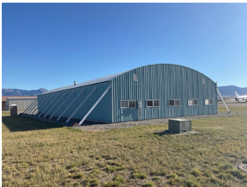
Figure 6.41. 24GA2320, Hangar 8, west corner, view to the northeast.
