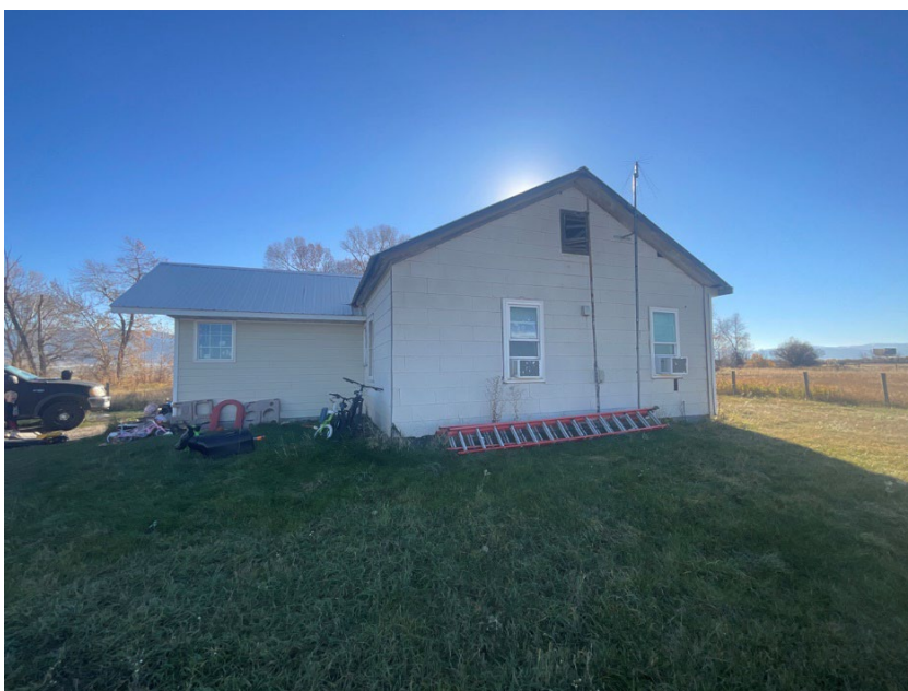
Figure 7.21. Feature 2 at Site 24GA0394, west elevation, view to the east.
