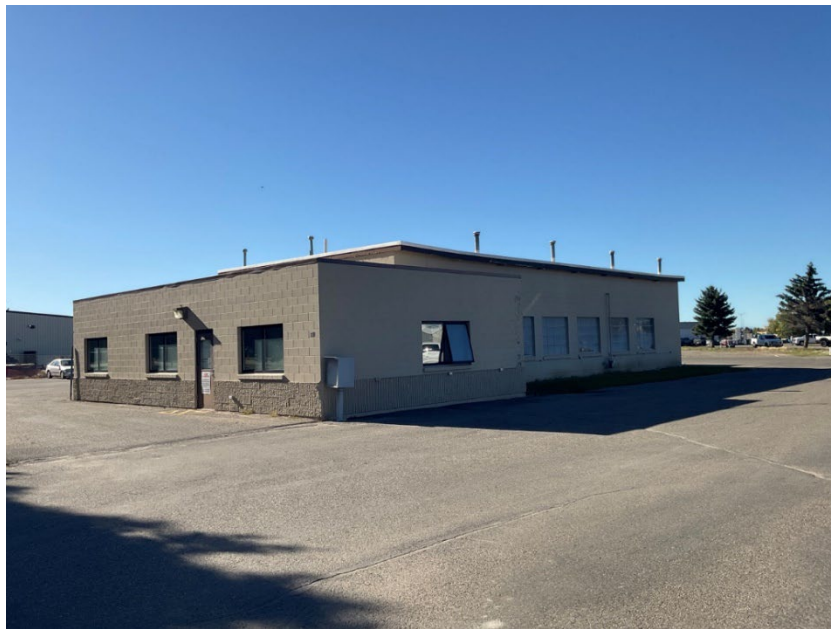
Figure 6.53. 24GA2316, east corner, view to the west.
