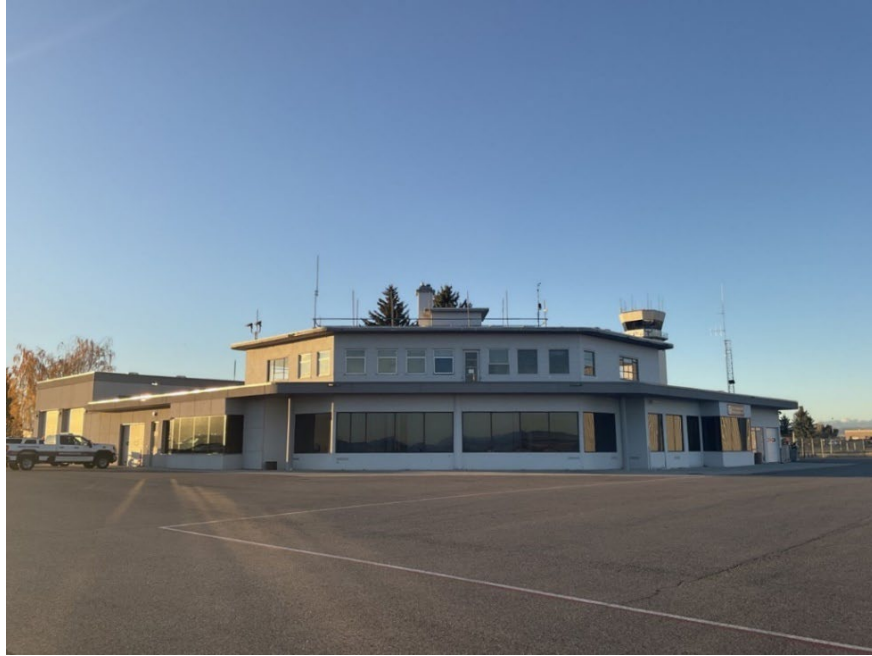
Figure 6.21. 24GA1654, north elevation, view to the south.
