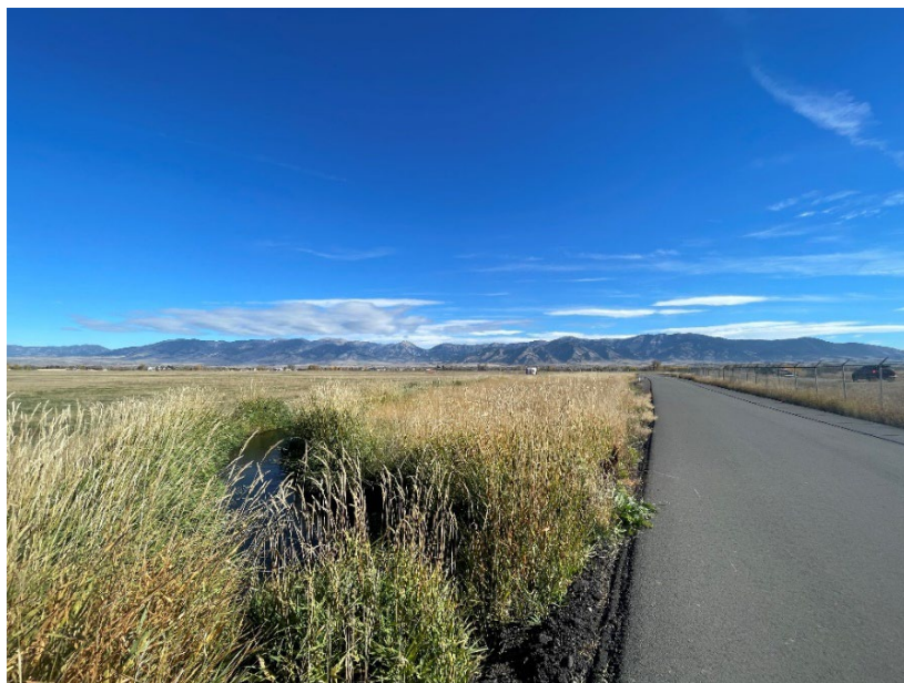
Figure 7.9. 24GA0743 at its crossing under Airport Road, view to the northwest.
