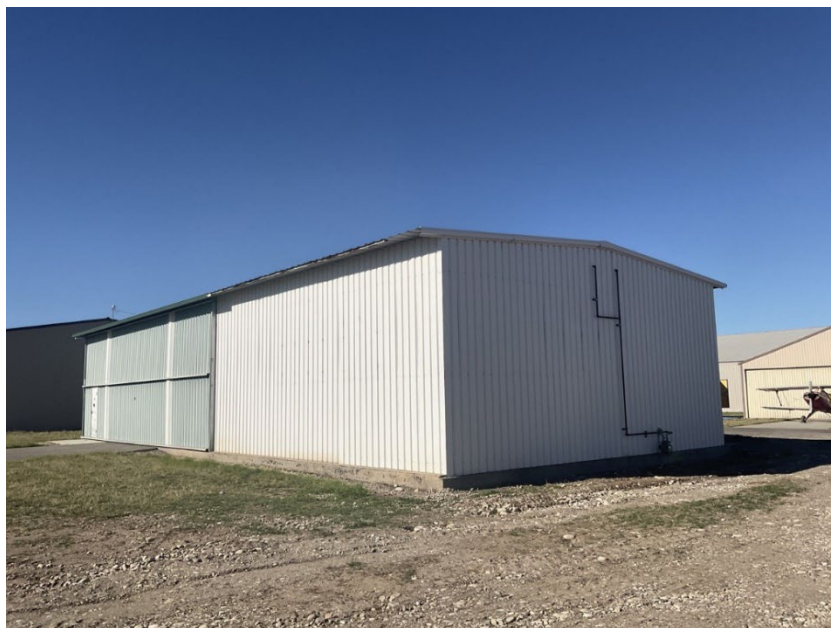
Figure 6.13. Hangar 28/39 from Taxiway J, view to the south.
