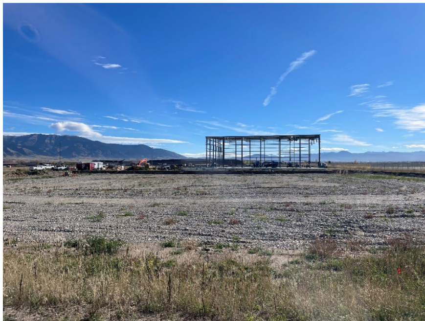
Figure 6.8. North Apron Flight School under construction, view to the east.
