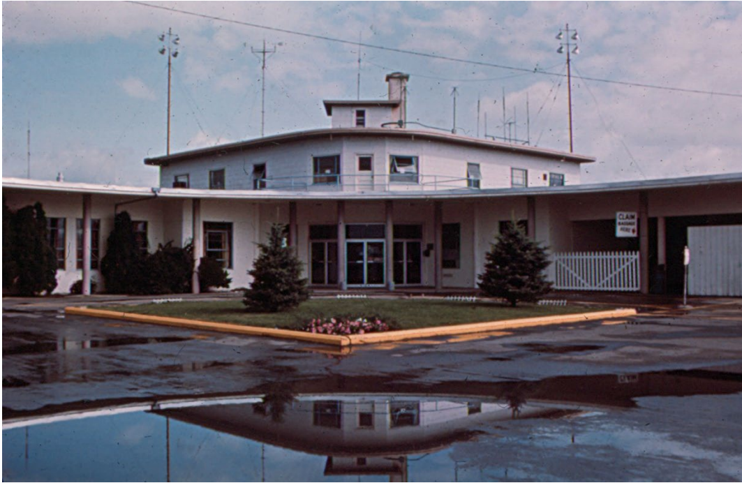
Figure 6.25. Circa 1976 photo of the terminal entryway, photo by Florence Shoebridge, courtesy of the Gallatin History Museum, Photo 16071-232.
