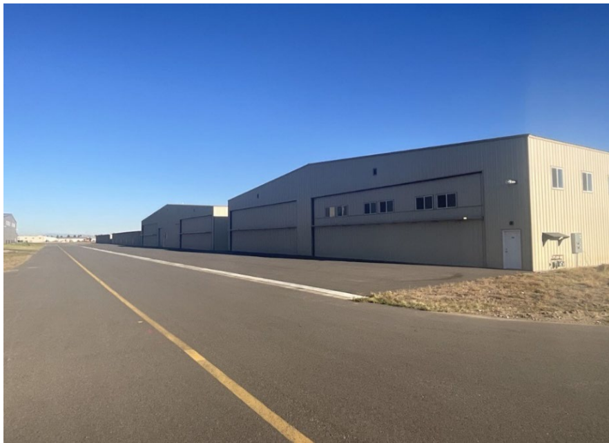
Figure 6.3. Modern hangars at Taxiway W from Taxiway X, view to the west.
