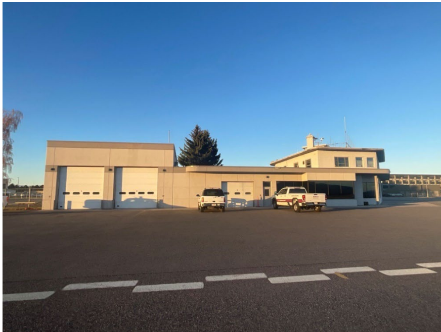
Figure 6.22. 24GA1654, northeast elevation, view to the southwest.
