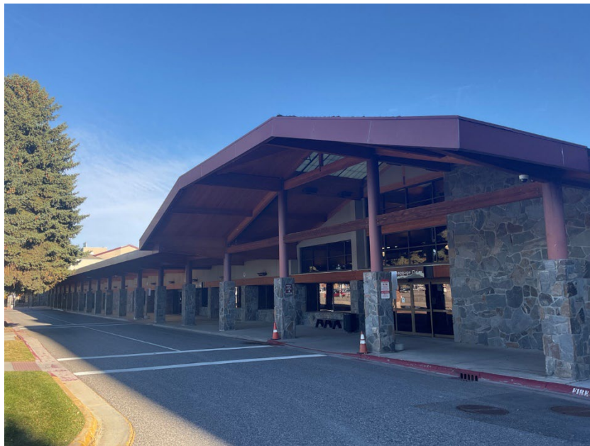
Figure 6.58. 24GA2343, entryway to the 1977 portion of the BZN terminal, now the ground transportation wing. View to the northwest.
