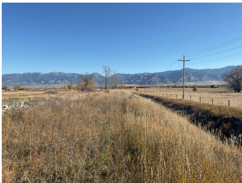
Figure 7.15. 24GA1096 railbed near Dollar Road, view to the northeast.
