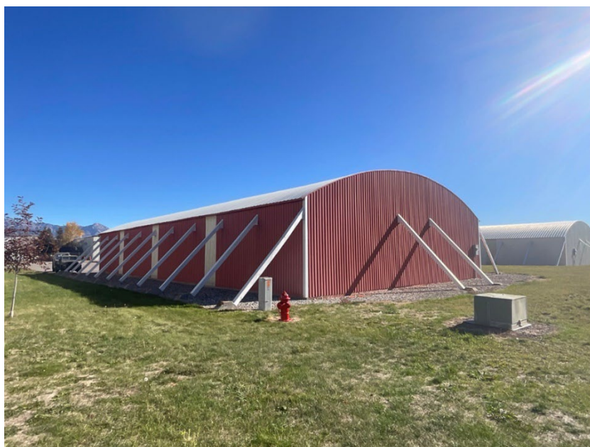
Figure 6.45. 24GA2320, Hangar 10, west corner, view to the northeast.
