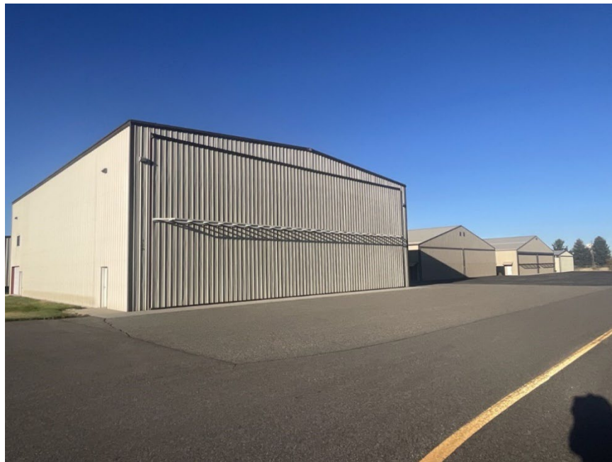
Figure 6.5. Modern hangars at Taxiway Q, West Apron, view to the west.
