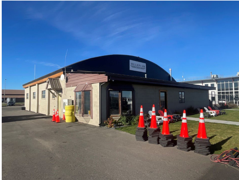
Figure 6.34. 24GA2319, east corner, view to the west.
