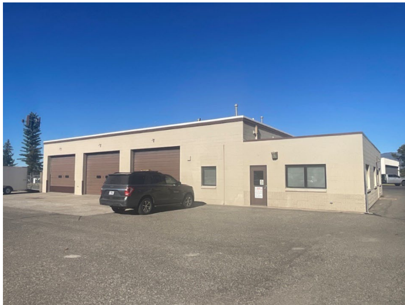
Figure 6.54. 24GA2316, southwest elevation, view to the north.
