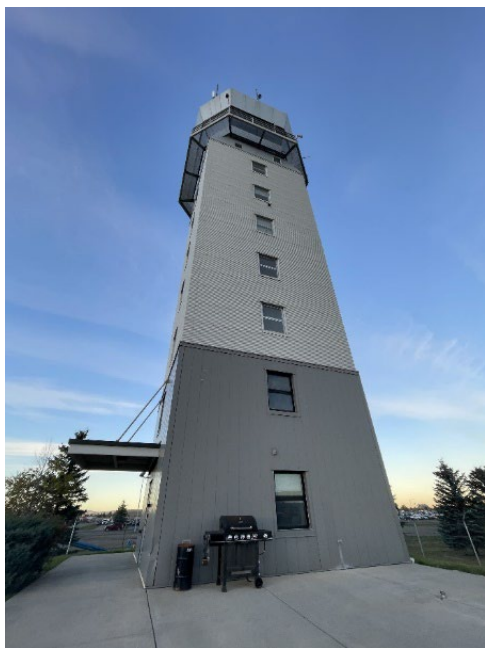
Figure 6.7. Modern (1997) control tower, view to the south.
