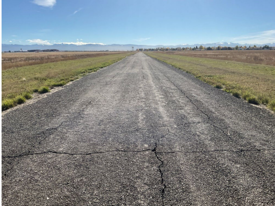
Figure 4. Overview of 24GA2317 from near Penwell Bridge Road, view to the south.
