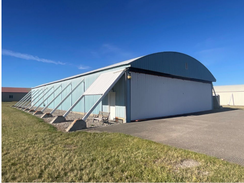
Figure 4. 24GA2320, Hangar 8, east corner, view to the west.
