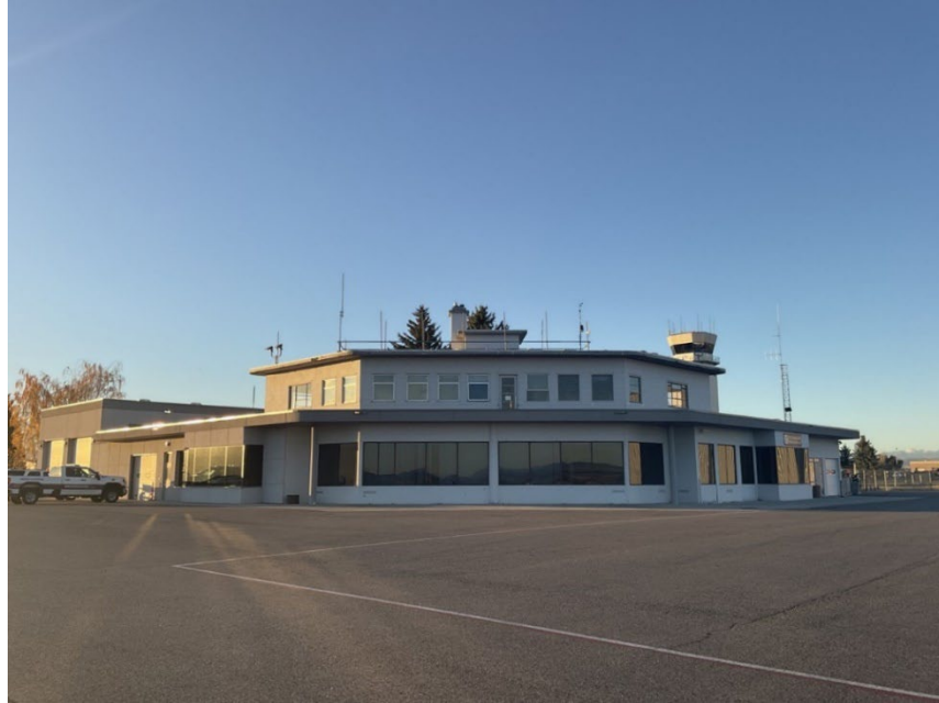
Figure 4. 24GA1654, north elevation, view to the south.
