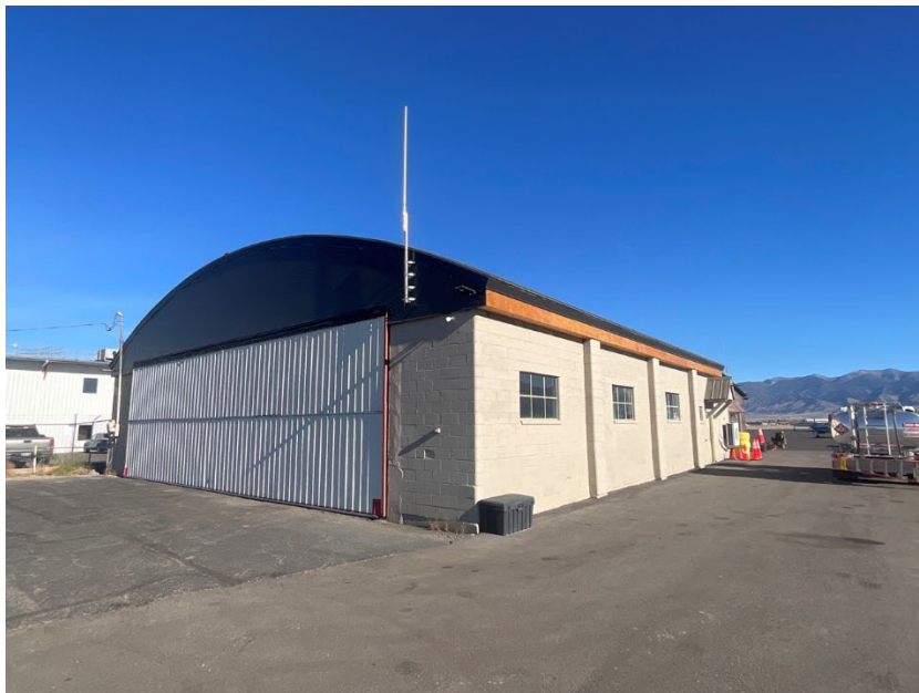
Figure 5. 24GA2319, south corner, view to the north.
