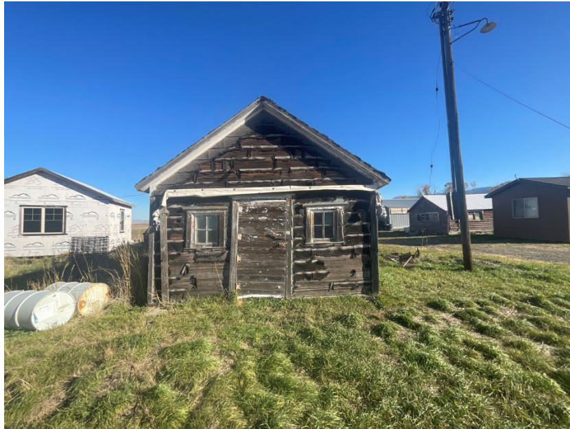
Figure 4. Feature 4 at Site 24GA0394, view to the north.
