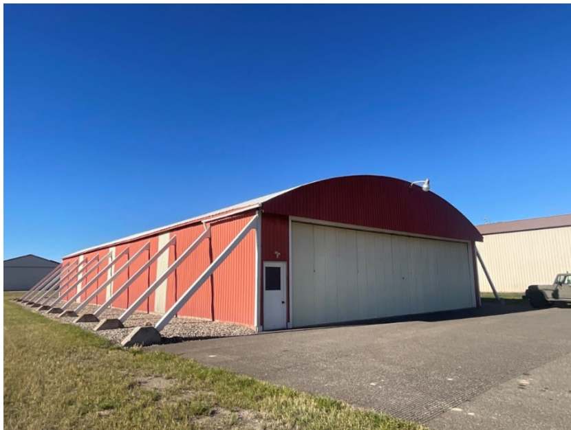
Figure 8. 24GA2320, Hangar 10, east corner, view to the west.
