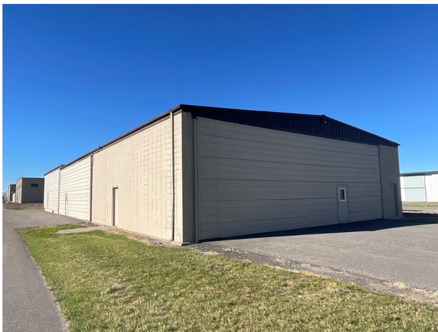
Figure 4. 24GA2318, north corner, view to the south.
