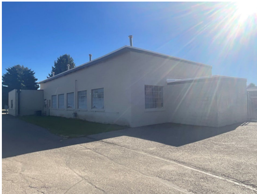
Figure 4. 24GA2316, north corner, view to the south.
