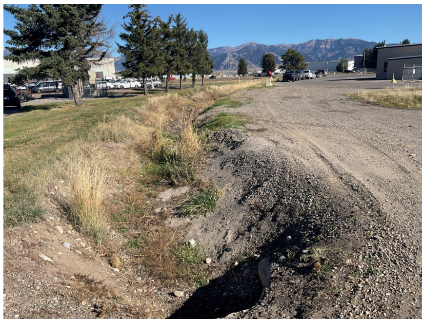
Figure 7. 24GA0743 abandoned segment west of Wings Way, view to the northeast.
