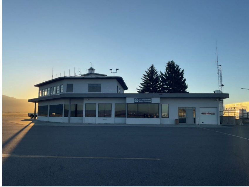
Figure 6. 24GA1654, northwest elevation, view to the southeast.
