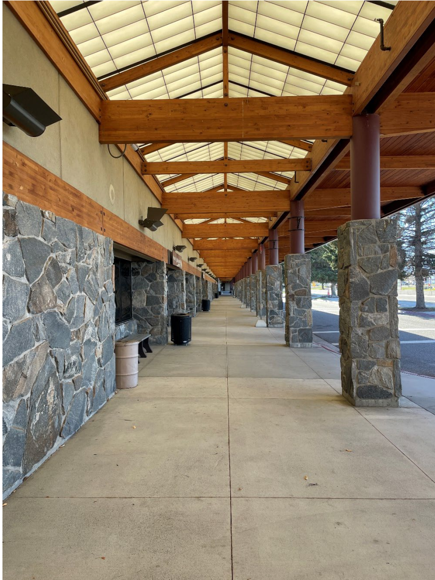
Figure 6. 24GA2343, existing 1977 rock work.
