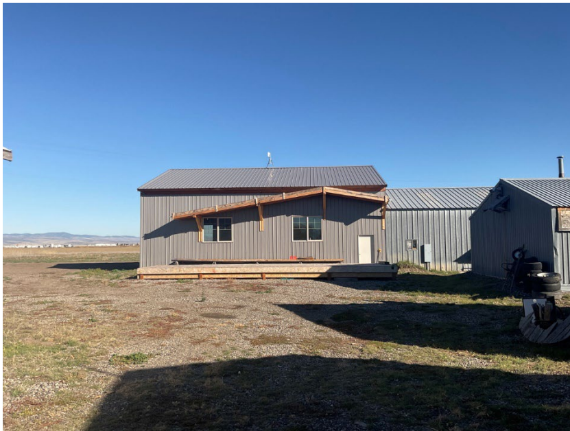
Figure 5. Feature 13 at Site 24GA0394, view to the north.
