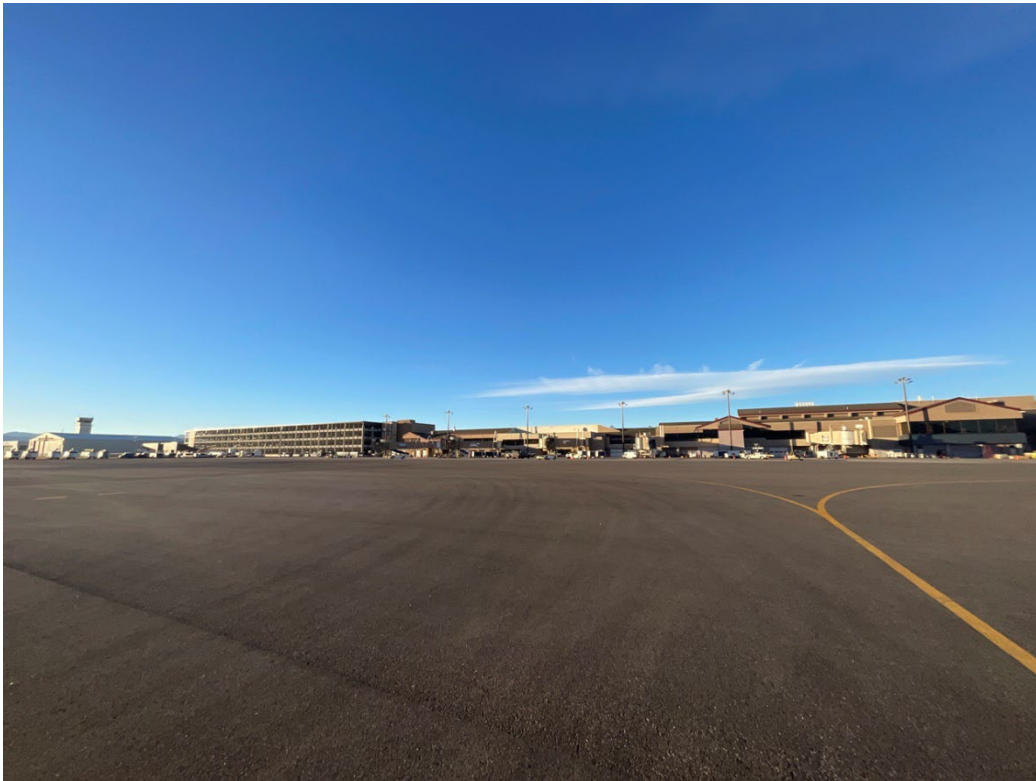
Figure 8. 24GA2343, overview showing the modern parking structure to the right, the 1977 terminal center, 1996 expansion to the right.
