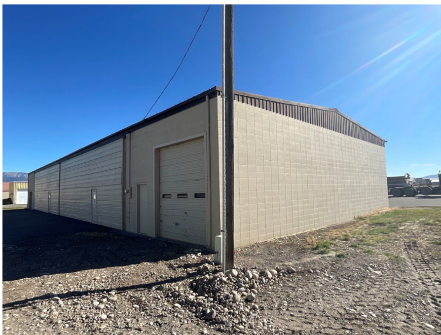
Figure 5. 24GA2318, west corner, view to the east.
