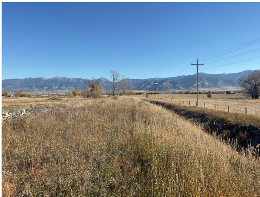
Figure 4. 24GA1096 railbed near Dollar Road, view to the northeast.
