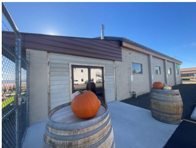
Figure 6. 24GA2319, north corner, view to the south.
