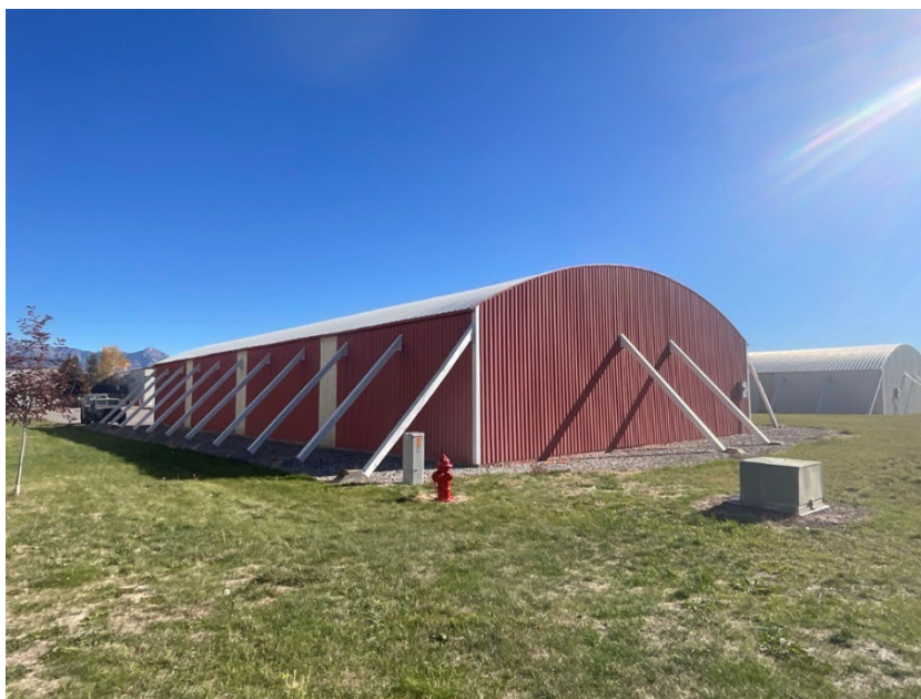
Figure 9. 24GA2320, Hangar 10, west corner, view to the northeast.
