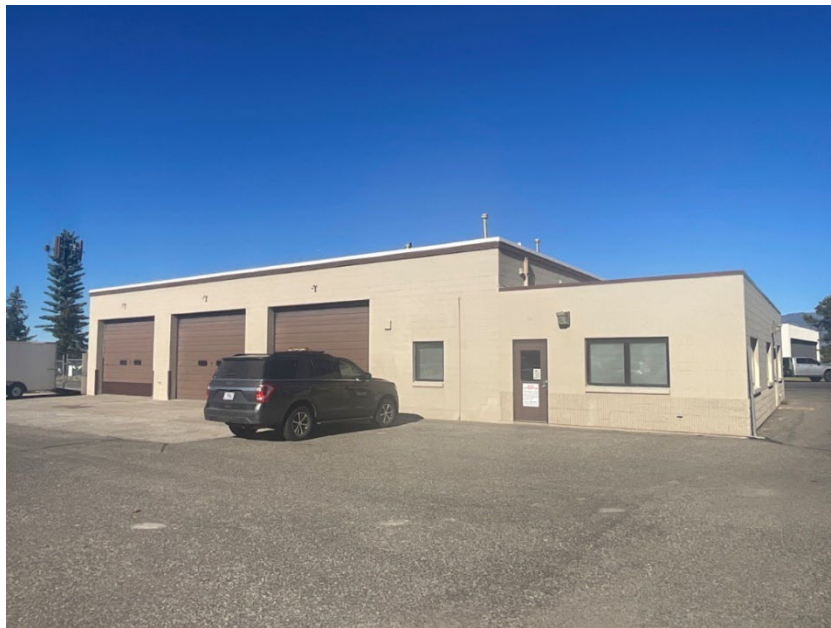
Figure 6. 24GA2316, southwest elevation, view to the north.
