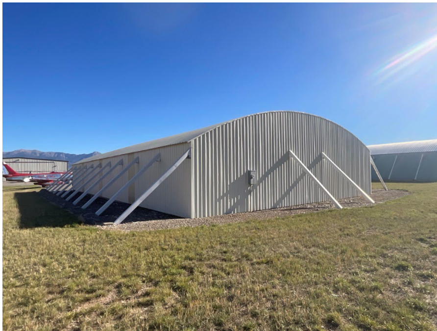
Figure 7. 24GA2320, Hangar 9, west corner, view to the northeast.
