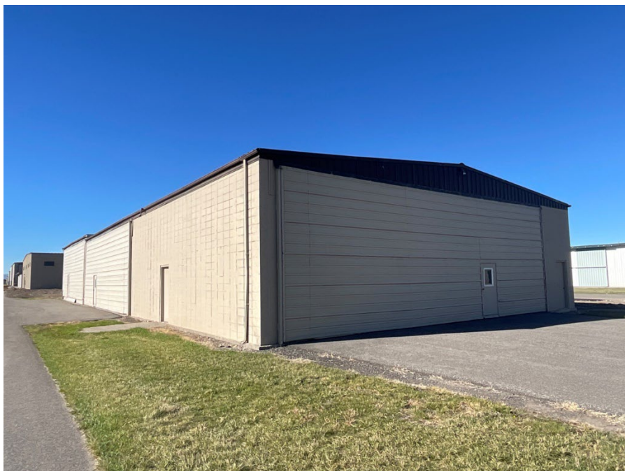
Figure 5. 24GA2318, north corner, view to the south.
