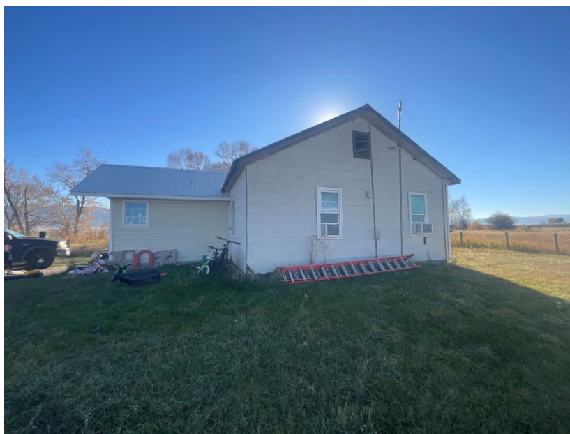
Figure 7. Feature 2 at Site 24GA0394, west elevation, view to the east.
