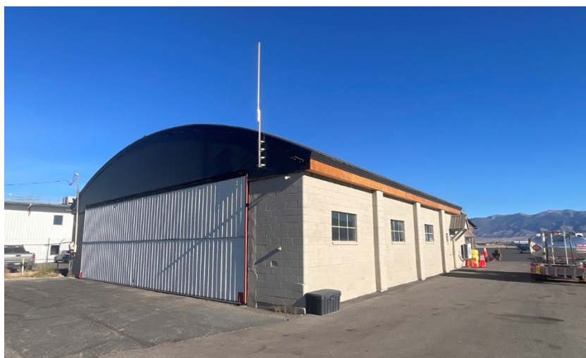
Figure 6. 24GA2319, south corner, view to the north.
