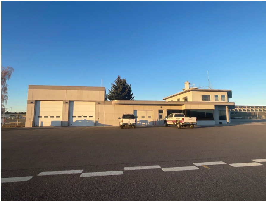
Figure 5. 24GA1654, northeast elevation, view to the southwest.
