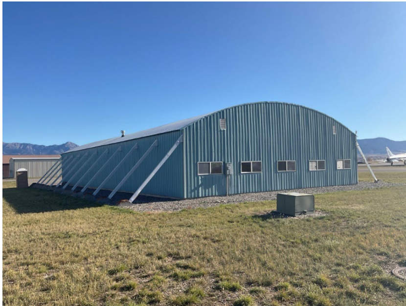
Figure 5. 24GA2320, Hangar 8, west corner, view to the northeast.
