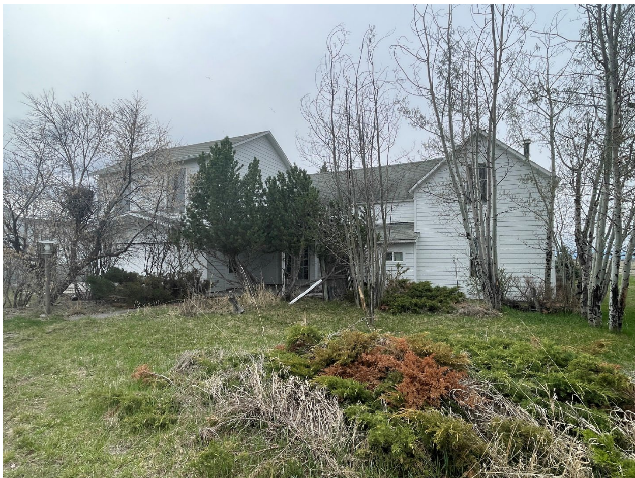
Figure 5. 24GA2327, north elevation, view to the south.
