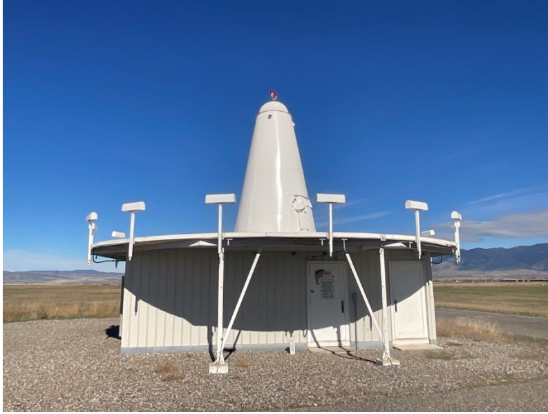
Figure 3. 24GA2322, the VOR at BZN, view to the north.
