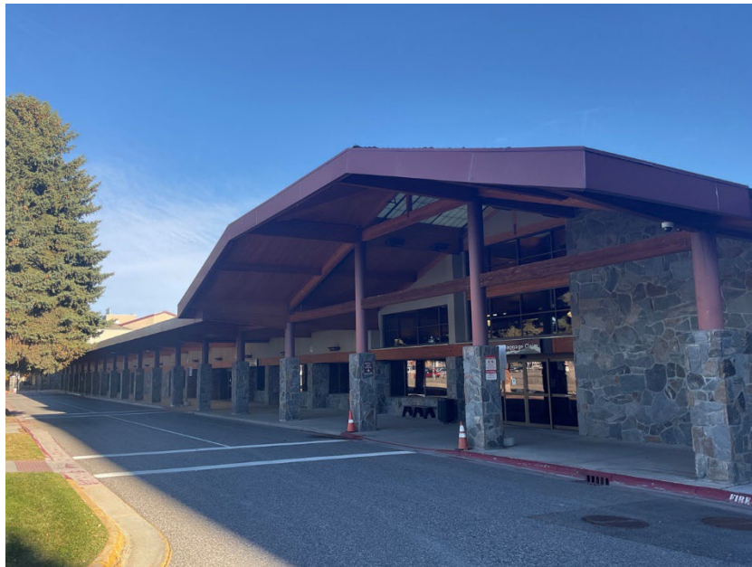
Figure 10. 24GA2343, entryway to the 1977 portion of the BZN terminal, now the ground transportation wing. View to the northwest.
