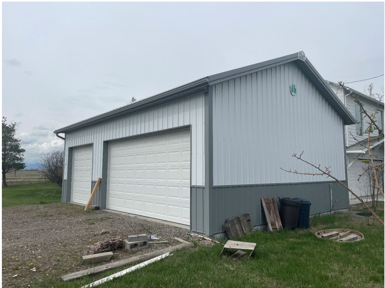
Figure 6. 24GA2327, modern shop, northeast corner, view to the south/southwest.
