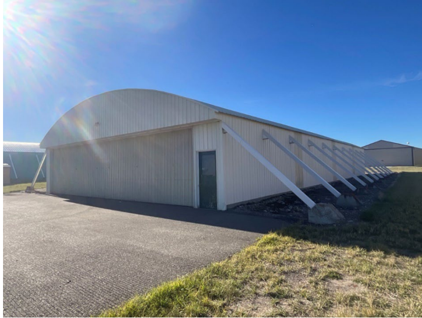
Figure 6. 24GA2320, Hangar 9, north corner, view to the south.
