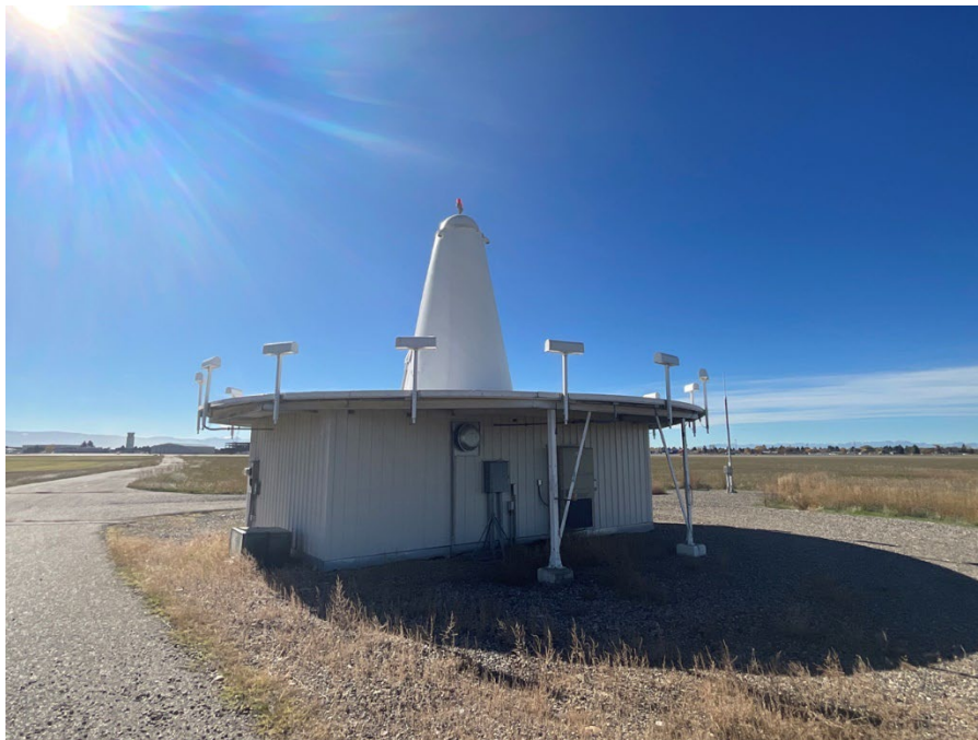
Figure 4. 24GA2322, VOR at BZN, view to the south.
