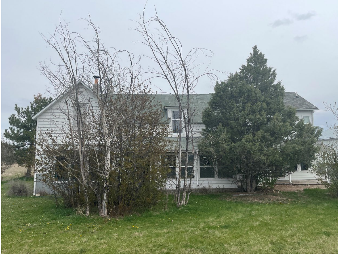
Figure 4. 24GA2327, south elevation, view to the north.
