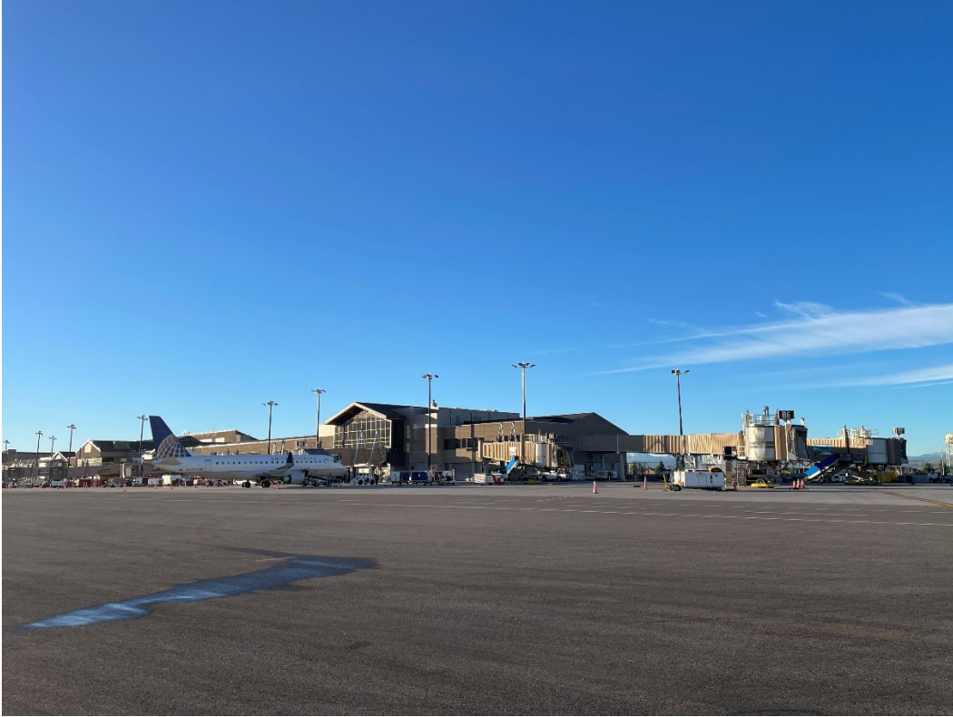
Figure 7. 24GA2343, modern Concourse B.
