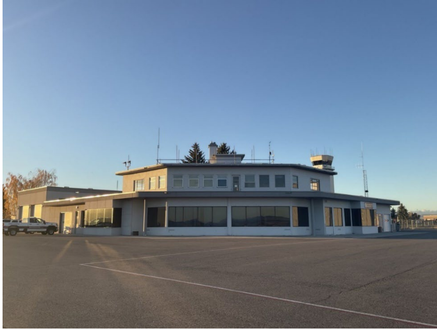
Figure 3. 24GA1654, north elevation, view to the south.
