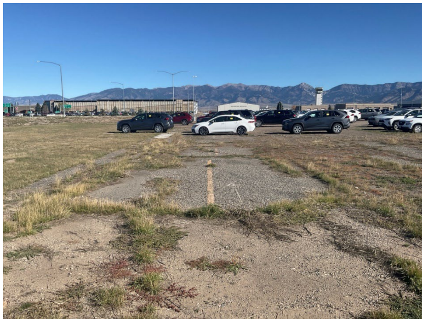
Figure 3. Taxiway "B" near its intersection with Airway Blvd., view to the north.
